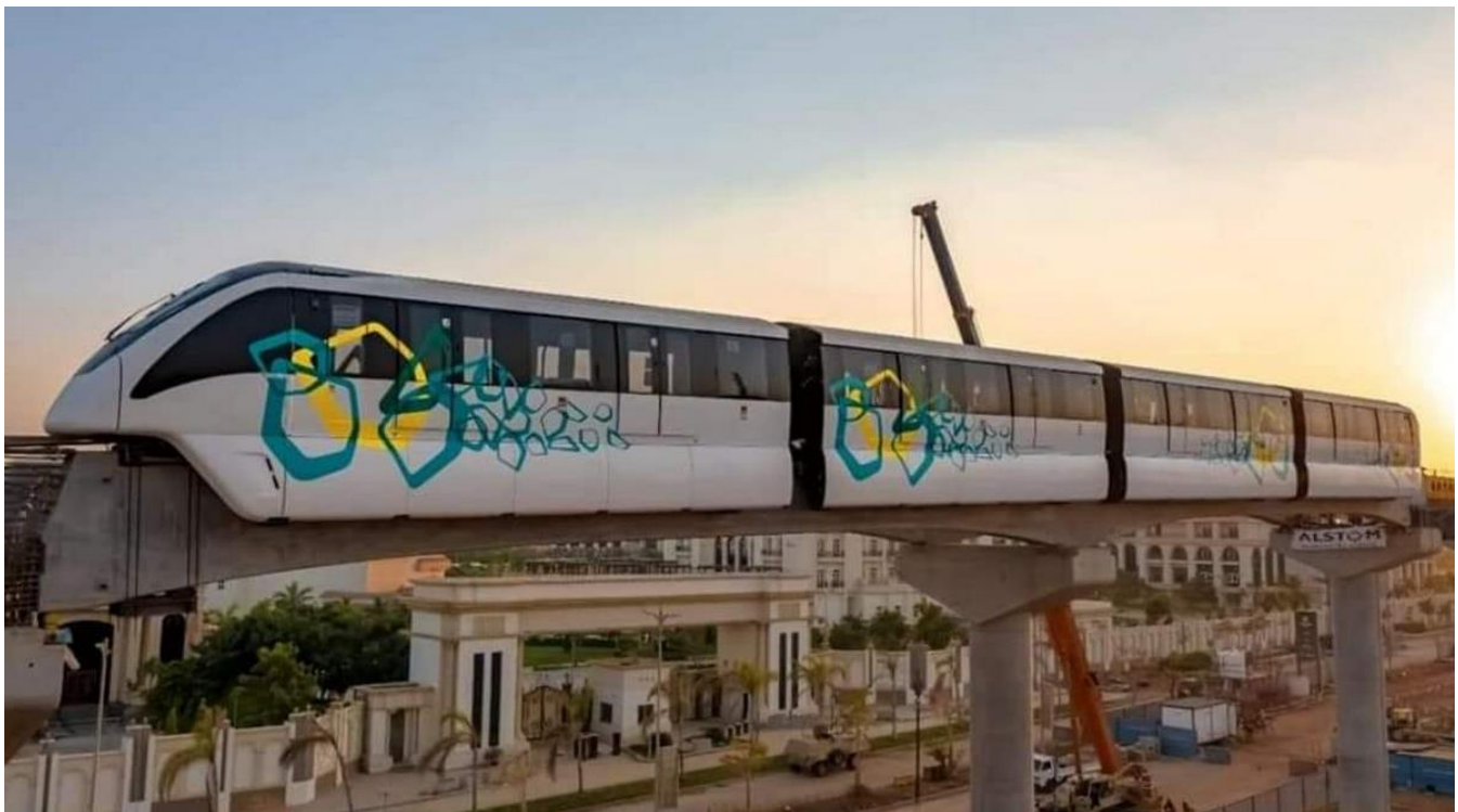
East of Nile Monorail (Quelle: National Authority for Tunnels)
