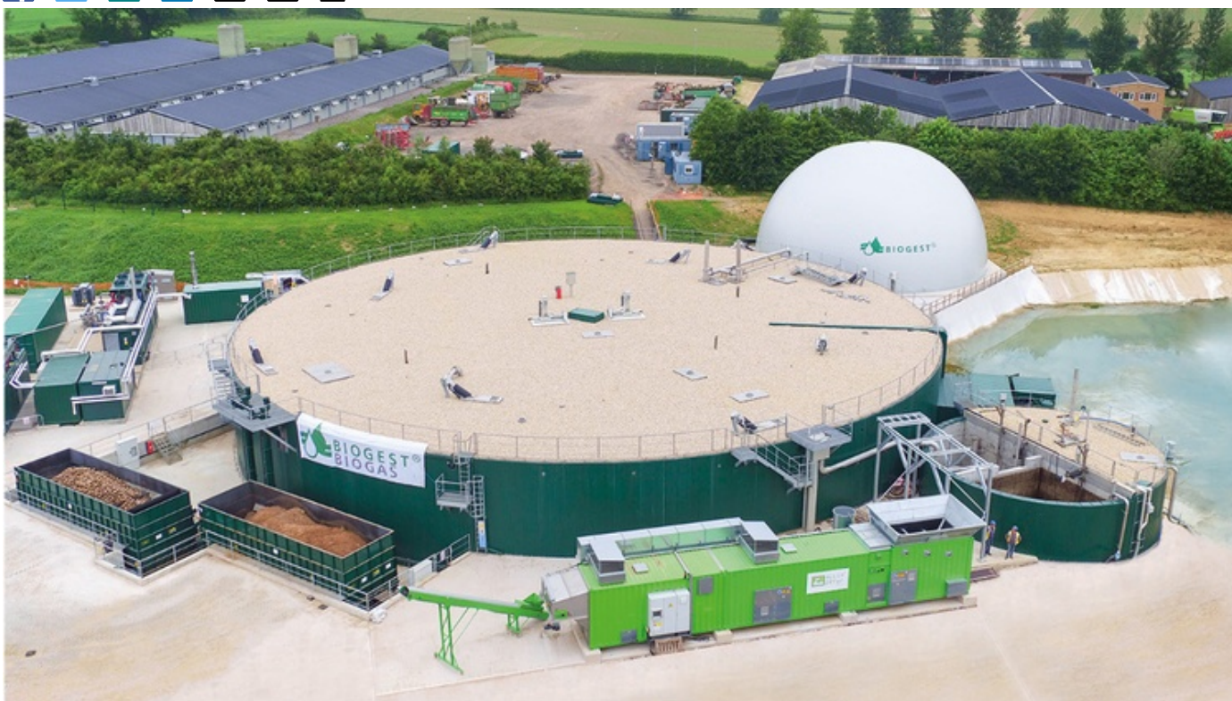
PowerRing Biomethaneinspeiseanlage Frogmary in UK
